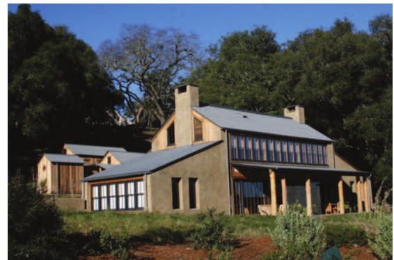
(b) final construction
