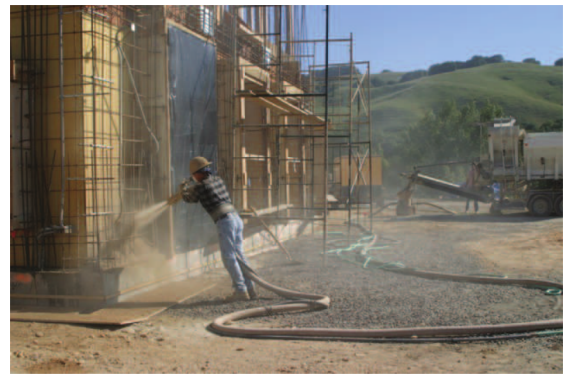
(a) work in progress
